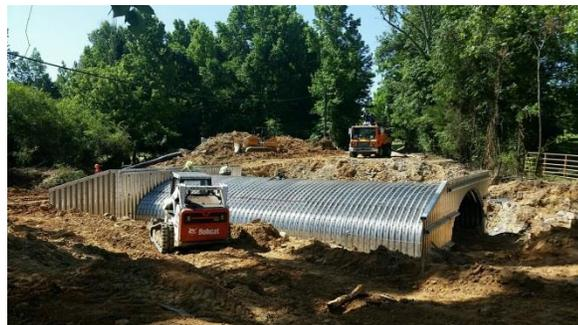
**Culvert being installed in stream channel**
