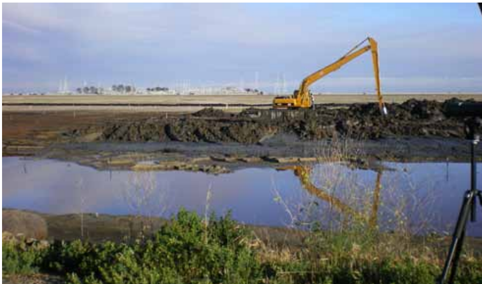
Construction at Pond SF2
