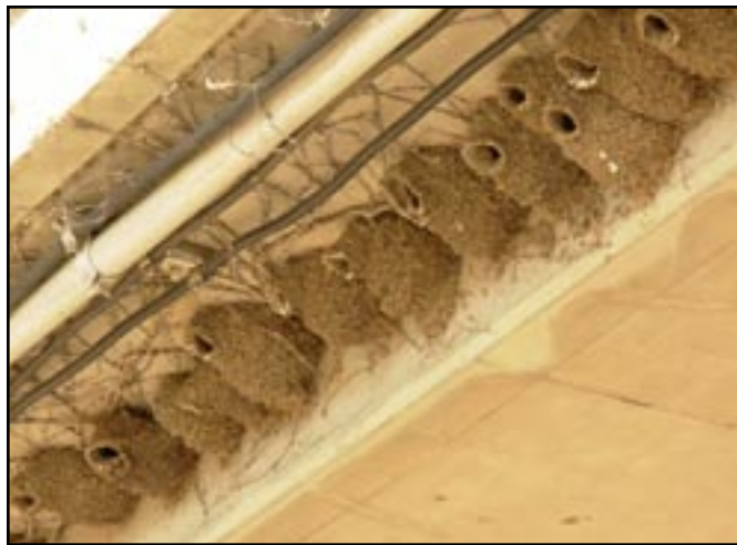
Cliff swallow nests on the underside of Dumbarton Bridge
