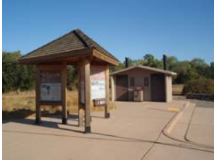
Information Kiosk & Restrooms
