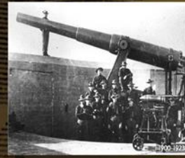
Fort Dade soldiers stand with "disappearing" gun at Battery Mcintosh. They called it a disappearing gun because the recoil made the gun drop down or disappear behind the wall for reloading.
