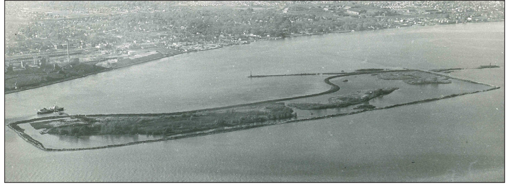
Grassy Island in 1962 showing the first perimeter dike constructed to contain contaminated sediments. USFWS
