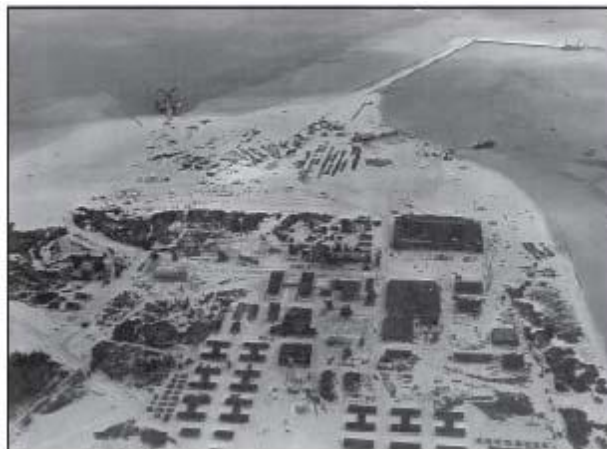
Figure 6. Aerial photograph of Midway Naval Air Facility at Sand Island under construction in 1941. (Navy)
