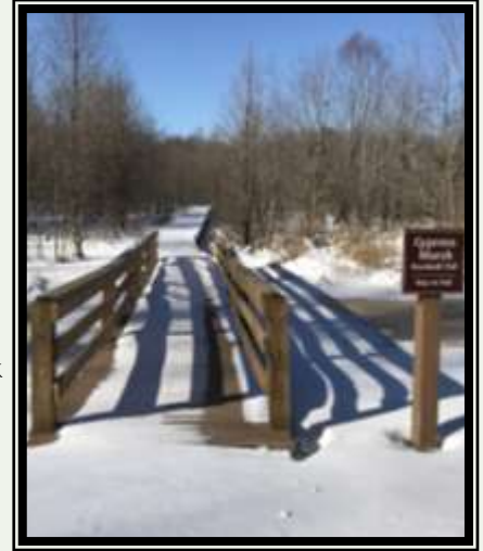
Boardwalk Trail Bridge over West Ditch
