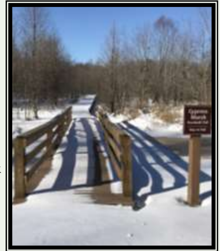
Boardwalk Trail Bridge over West Ditch
