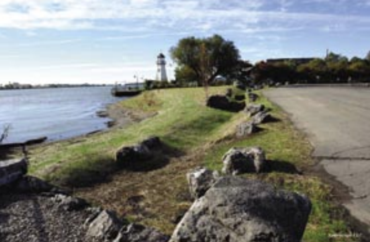
Before-and-after photos showing soft engineering techniques at DTE's River Rouge Power Plant, Nativescape
