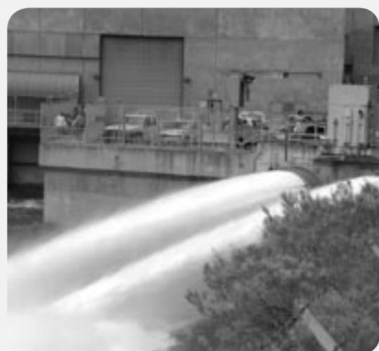
AT FLAMING GORGE DAM WATER RELEASES THROUGH TUBES THAT BYPASS THE POWER PLANT MAY BE NEEDED TO HELP ACHIEVE FLOW CONDITIONS FOR ENDANGERED FISH AS DESCRIBED IN THE RECORD OF DECISION.
