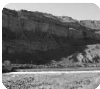
A FISH PASSAGE IS SLATED FOR 2007 AT THE PRICE-STUBB DIVERSION DAM.
