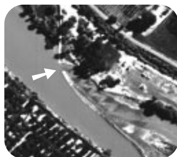
A FISH PASSAGE (SEE ARROW) CONSTRUCTED AT THE GRAND VALLEY IRRIGATION COMPANY DIVERSION DAM AND CANAL BECAME OPERATIONAL IN 1998. THE FISH SCREEN BECAME OPERATIONAL IN 2002.
