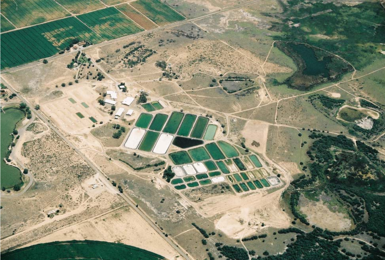
Aerial Photo of Dexter National Fish Hatchery & Technology Center 2004 Photo courtesy of Dr. Robert Flynn, NM State University – Agriculture
