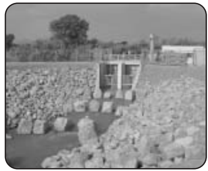
Fish passage at Public Service Company of New Mexico weir.
