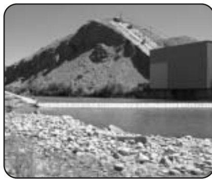
Arizona Public Service Company weir.
