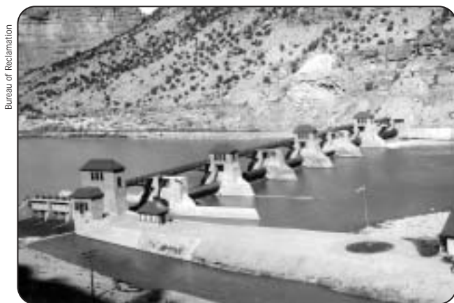
The Grand Valley Project Diversion Dam was completed in 1916.
