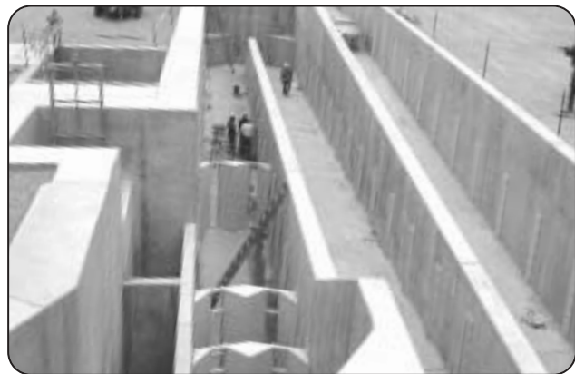
The new fish passage under construction in May 2004.
