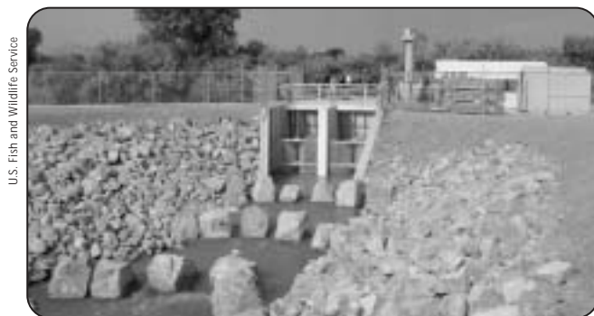
Endangered fish continue to use the fish passage opened in 2003 at the Public Service Company of New Mexico Weir.
