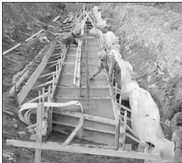
A fish passage structure at the Public Service Company of New Mexico Weir will be completed in 2003. Fiscal Year 2004 funds will be used to design a fish passage at the Arizona Public Service Weir.
