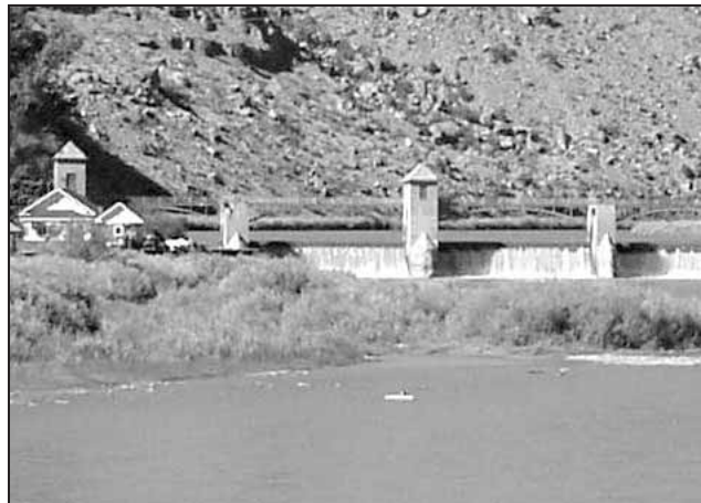
Construction is slated to begin in 2004 on a fish passage for the Grand Valley Project Diversion Dam near Grand Junction, Colorado.
