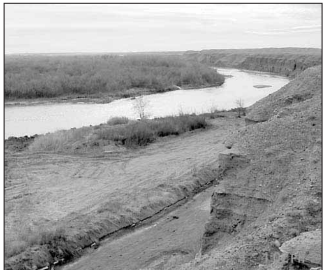
Removal of the Cudei Diversion Dam on the San Juan River improved habitat for endangered fish by restoring the natural channel. A stub of the dam was left in place to prevent erosion.
