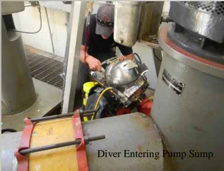
Contractor, Inland Potable Services, completed the intake water line gate closing project. The solution to close the gate after the evaluation was to cut the stem and seat the gate in the wedges, permanently closing the opening. WBNFH is now flowing water through the upstream intake pipeline only.
