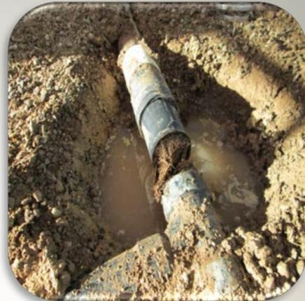
Drainage Issue, pipe filled with tree root
