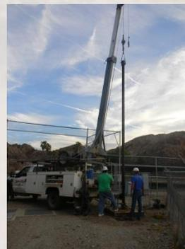
cause of reduced water flow. A small hole was located the pump pipe. The pipe was replaced, the well screens scrubbed, the pump and motor pressure washed and reinstalled.
