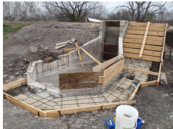
Framing for concrete steps and kettle repair
