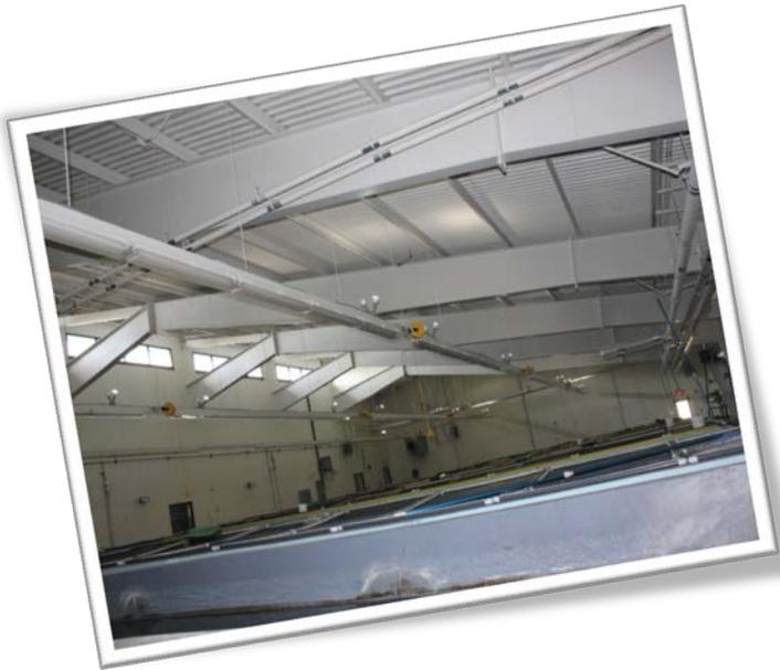
The automatic lighting system that maintains the diurnal light cycle in the hatchery building failed during the latter part of December. The company that installed and constructed this system has been out of business for approximately 15 years, making efforts to simply find replacement parts impossible. The system had to be operated manually since the failure. The cost of rehabilitating the old system exceeded that of
