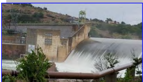
This is what recent flooding has done in the central Texas area. Water has been going over the entire length of the spillway at Inks Dam now for two and half weeks.
