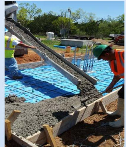
Work being performed for the new generator pad. Once completed this generator will protect the two production wells used for shipping fish throughout Region 2 and the Endangered Clear Creek gambusia.
