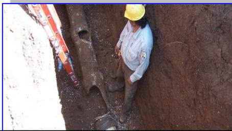
Above: Once we found where the pipe was leaking it became obvious that expensive repairs were needed and assuming they all were repaired this way, more to come! Please note the hose clamps holding the rubber gasket onto the pipe. Below: Done correctly and longer lasting but more expensively.
