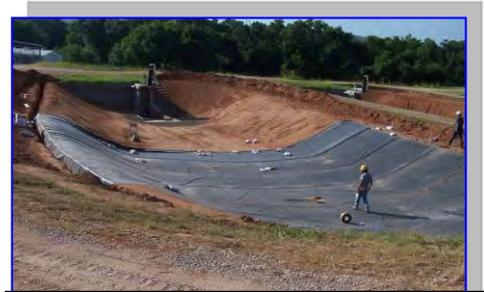
EPDM liner being installed in one of the early rearing fry ponds. These save on water, chemicals and labor costs.
