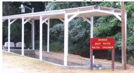
The raceway cover is an all-welded frame and roof over raceway 1 for the mussel program. This will allow for security for endangered species and have the ability to use natural water for these delicate species.
