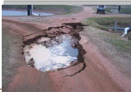
This is the creation of a new pond caused by the lateral line break servicing the 5, 6 and 7 series ponds. An additional two breaks were found going to ponds 5A and 6B.
