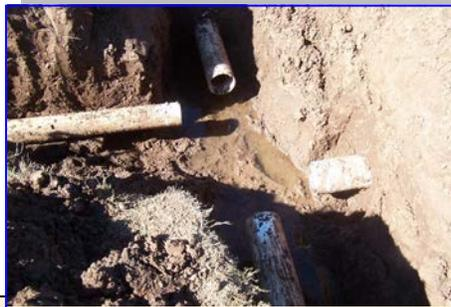
The intersection, were the breaks occurred, feeding incoming water to the 5, 6 and 7 series ponds. Unfortunately these pipes were 8 inch pipe when the ARRA Project contractors installed them so parts were special order.
