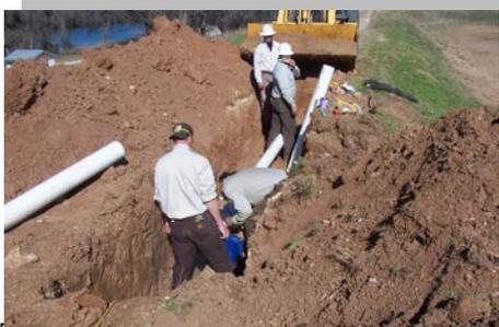
Hatchery staff repaired the line break on the 13 series of ponds and then replaced an “old” gate valve to a newer butterfly valve on pond 13B.
