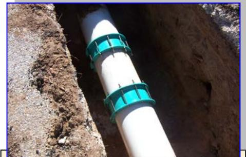
Completed repairs on the 16 inch drain line. Industry experts suggest that when it was installed it was pushed on too hard with a backhoe and split the bell end. When the incoming water line broke that serviced the eight ponds feeding into to this line, it filled it completely, and showed us where it leaked.
