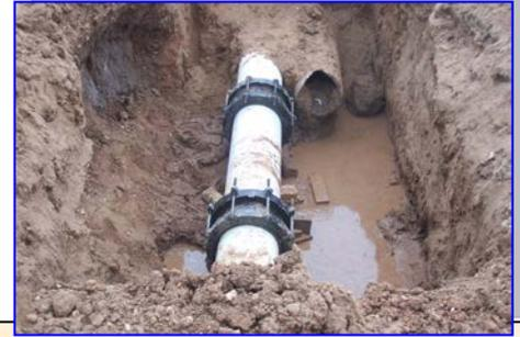
An incoming water line where for some reason new pipe was spliced into new pipe and the couplers failed. These pipes (pictured above) are 12 inch lines that fed five ponds but 8 inch pipe was used for eight ponds in a prior repair. Note the old pipe still left in ground.
