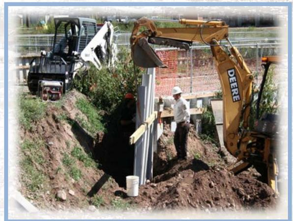
*Left: Effluent control structure taking shape for concrete pour. Above: Securing sheet pile together with support beams*
