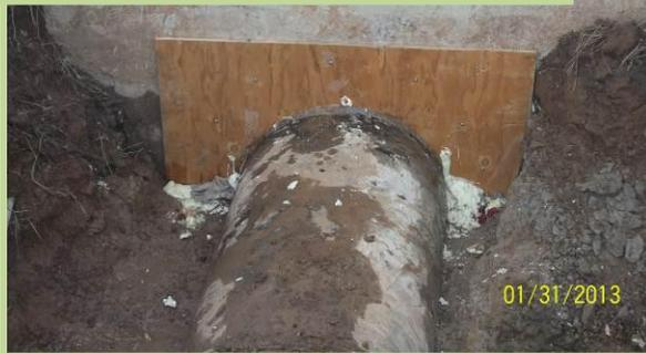
Fish friendly hydro-active expansion grout was used to seal the pipe leak at the water control structure
