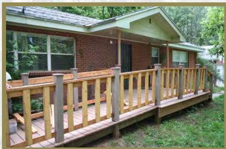
Jimmy Smith and Pete Drevnick began the task of replacing the old trex railing on the front porch of the Arizona Fish and Wildlife Conservation Office (AZFWCO) at the Alchesay NFH, that was damaged from a large willow tree branch during a wind storm and restoring it with old fashion wood boards. The wood boards were treated with an undercoat sealant and stained to prevent it from deteriorating.
