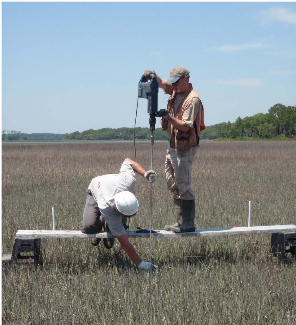
Installing SET Benchmark - Pinckney Island
