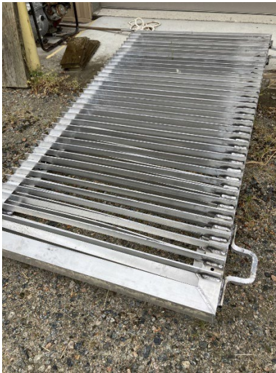
Figure 11. At least one carp barrier at each tide gate (4 total) have been cut in half to reduce the weight of lifting during high water flows for debris passage. The lower half of the gate remains in place and the upper half is lifted.
