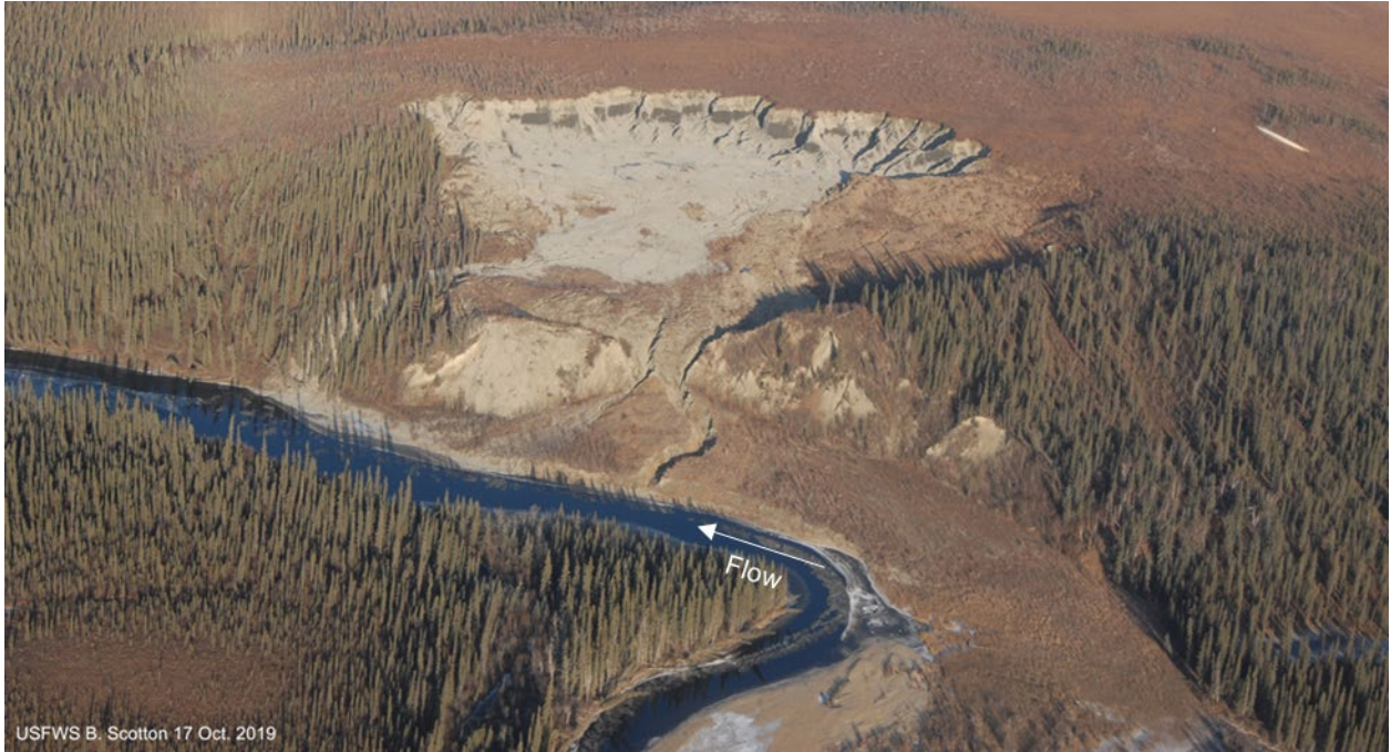
Figure 19. —An October 17, 2019, slump reconnaissance photograph. Note the newly exposed perimeter headwall bearing ice-rich soil that thawed and flowed down through a new outlet chute just downstream of the original outlet. The right-hand third of the slump persisted as evidenced by the established vegetation on the original slump floor. See Figure 4 for a comparison to the slump's condition in July 2018.
