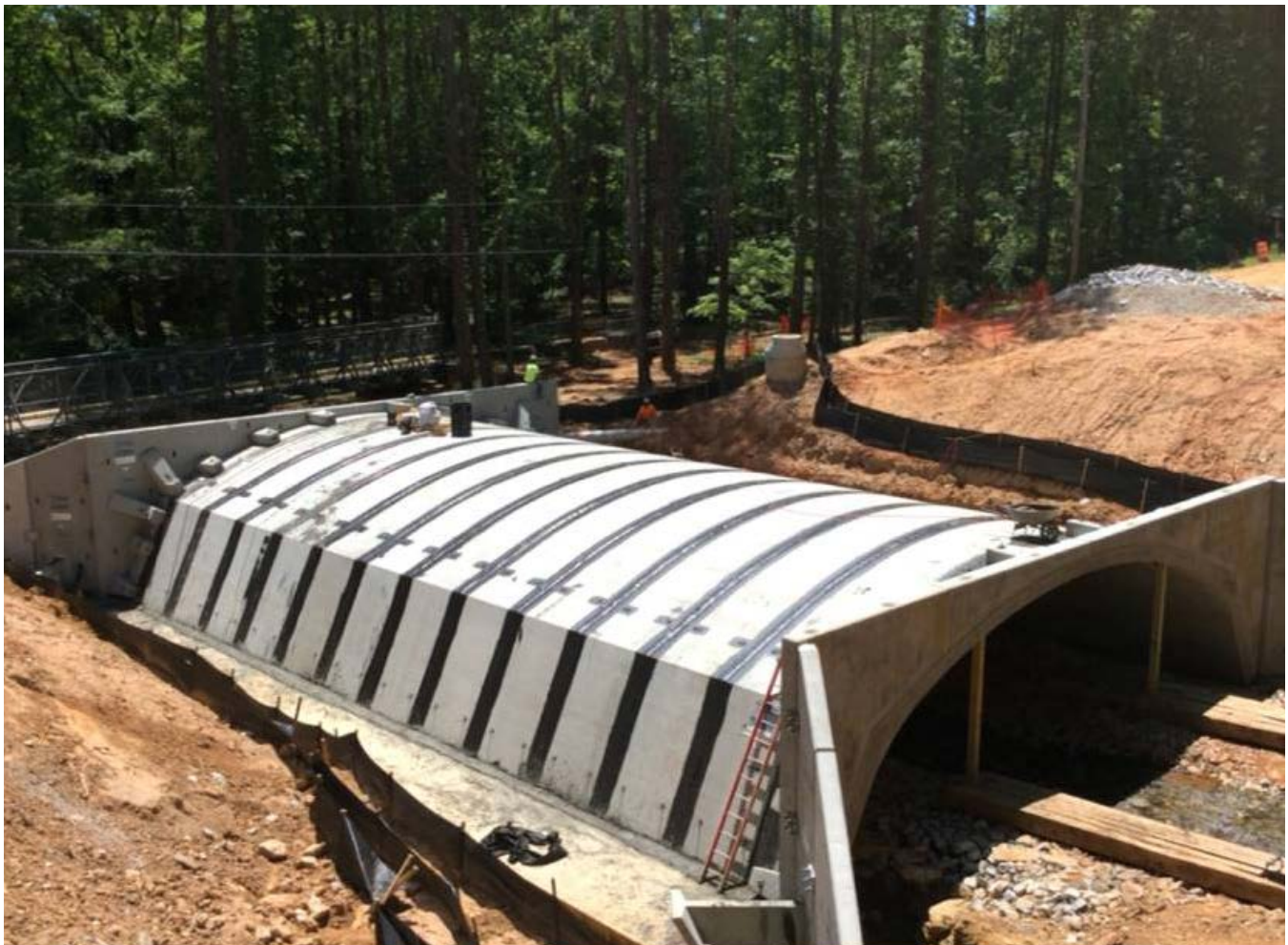
Concrete bottomless arch culvert being installed in Kedron Creek in Fayette County, funded by a SPLOST in 2017. Credit: Fayette County Road Dept.
