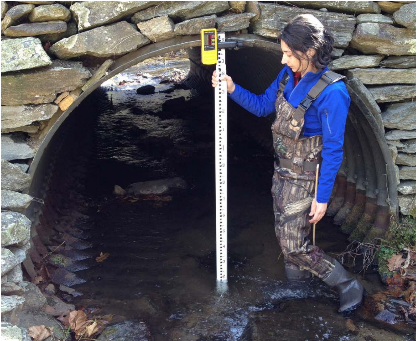
Field technician measures the height of a metal pipe culvert. Credit: Duncan Elkins/UGA
