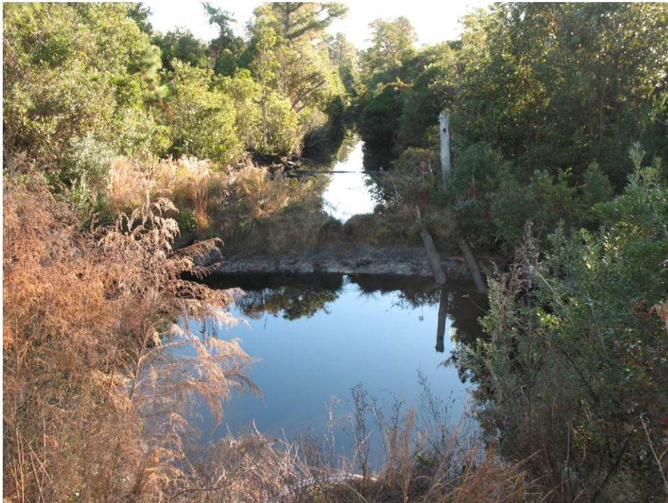
Figure A-29. Earthen plug, built with hand tools, on the far side of J Canal.
