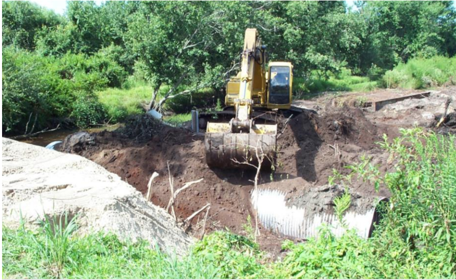
Figure A-14. Culvert installation.
