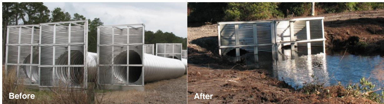
Figure A-11. Flashboard riser water control structures, before and after installation.
