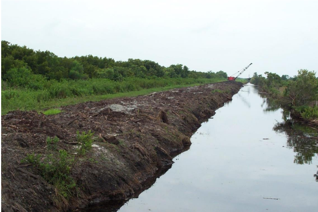
Figure A-10. Canal maintenance with excavated material placed on top of adjacent dike.
