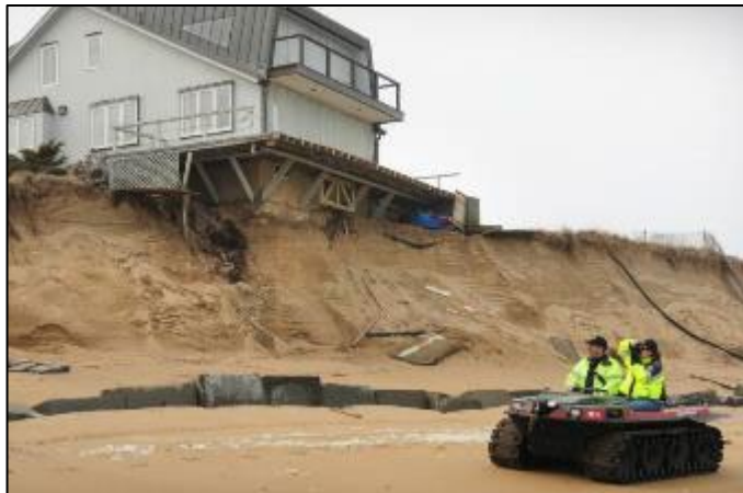
Photo 2-6 Coastal erosion occurring near Plum Island Center, Newbury, MA in April 2013. Credit: Bryan Eaton, Newburyport Daily News.
