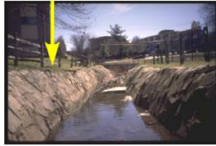
Poor Range (MD Save Our Streams) (arrow pointing to channelized streambank with no vegetative cover)
