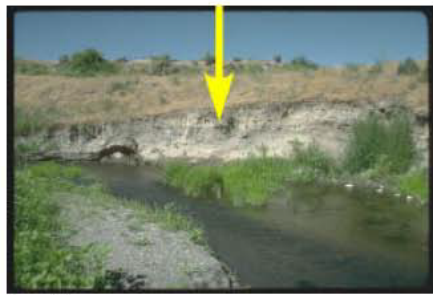
Poor Range (arrow highlighting unstable streambanks)
