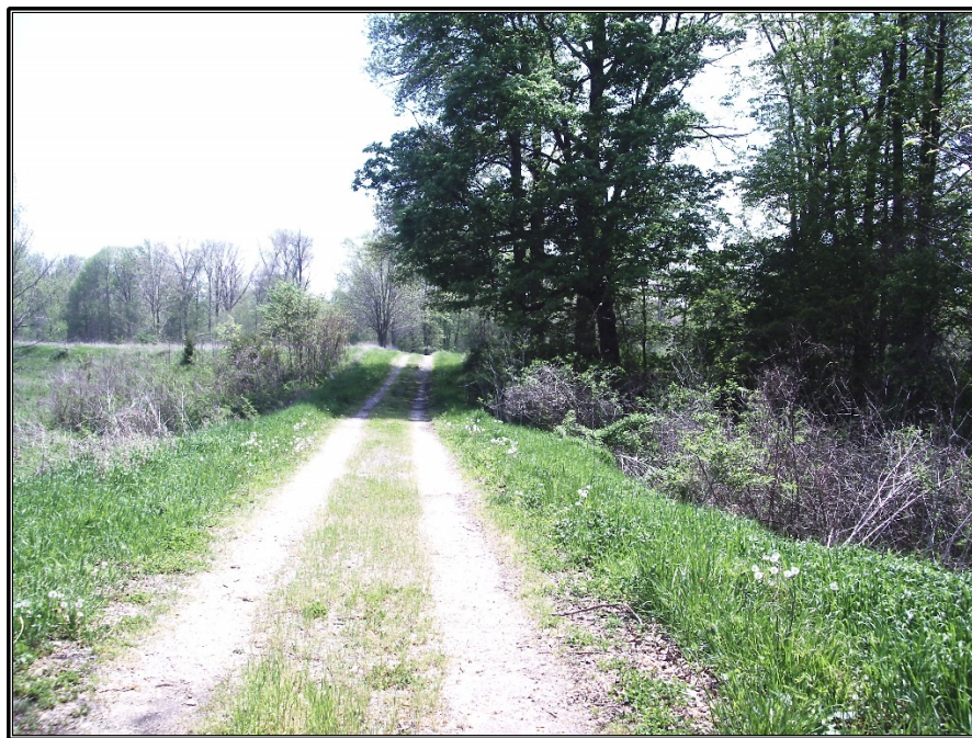
Figure 7. Overview of unimproved gravel road on western boundary, facing south.
