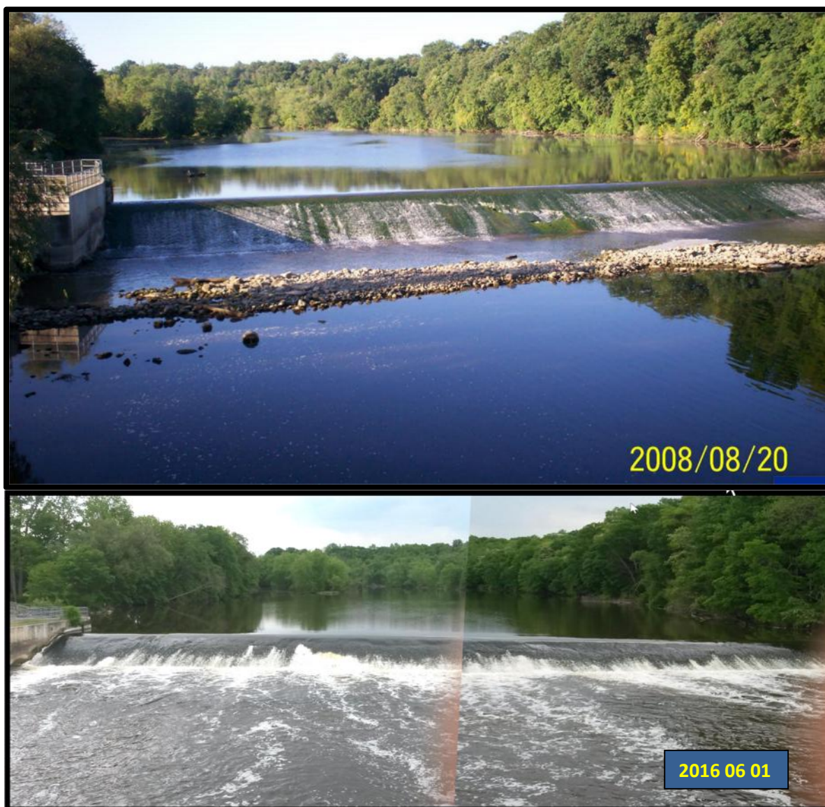
Figure 1. Face of Lyons Dam about 8 years apart.
