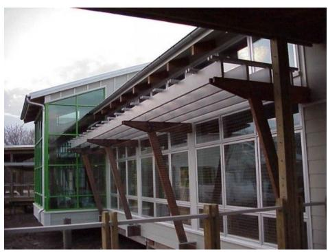
Netting installed on slanted wooden beams. Photo by USFWS.
