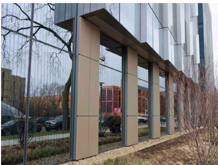
Paracord treatment on University of Chicago glass. Photo: Acopian BirdSavers
