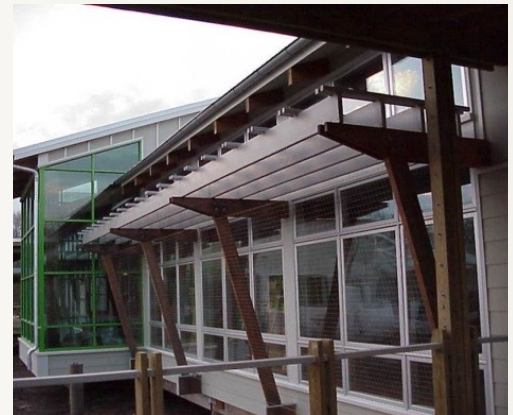
Netting installed on slanted wooden beams. Photo: USFWS
