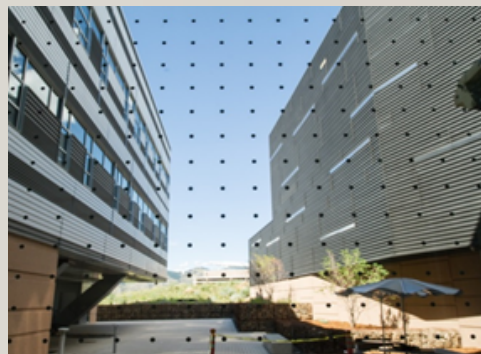
Dot pattern applied to exterior of National Renewable Energy Laboratory (NREL). Photo: Dennis Schroeder, NREL 31193
