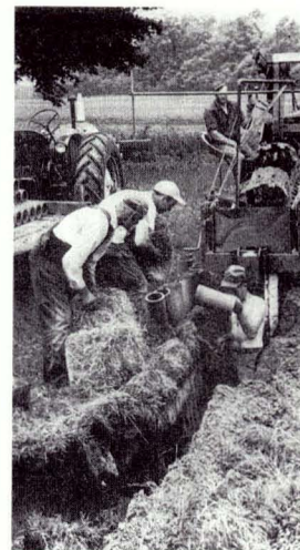
Drainage tile operation, circa 1940's. Tiles provide a conduit for moving water from a wetland. (Photograph courtesy of U.S. Department of Agriculture.)
