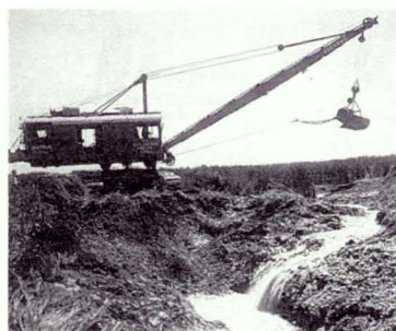
Oil-powered dredge digging a 30-foot-wide ditch to drain wetlands near Carroll, Iowa. (Photograph courtesy of National Archives, 8-D-2214-2570.)
