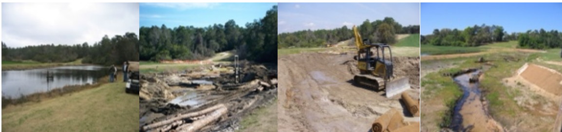
Figure 2. The phases of stream restoration in an Okaloosa darter stream through the Eglin golf course. From left: prior to restoration, pond drained and muck removed, floodplain established, stream channel created. Okaloosa darters naturally colonized this project within six months of completion.
