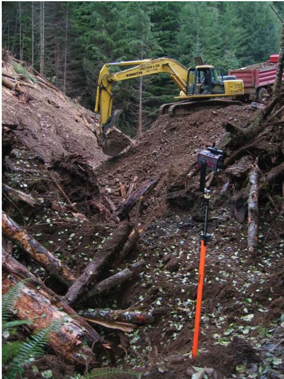
Excavator recontouring at a stream crossing road removal site
