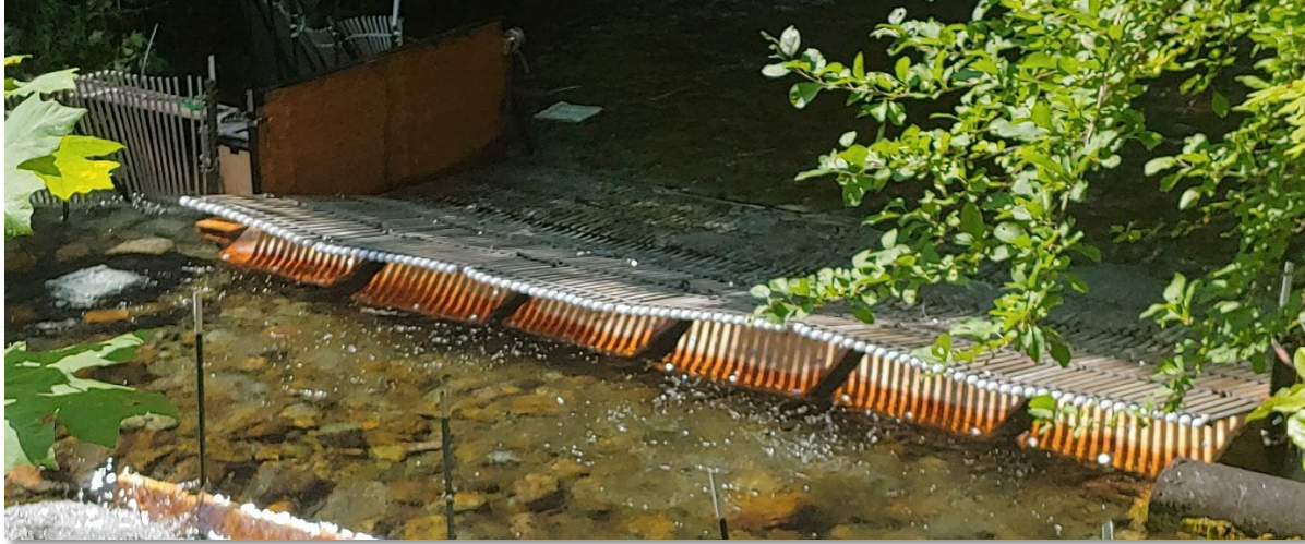
Figure 3. Photo depicting the aluminum picket leads, resistance board weir panels, video chute and camera chamber deployed in Cougar Creek.
