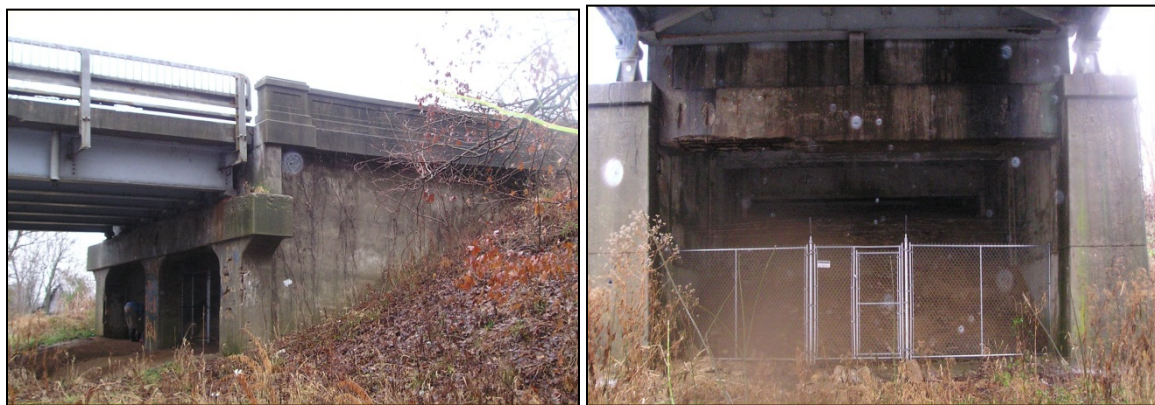
Photo 12 and 13: Bridge design mimicking “cave-like” atmosphere
