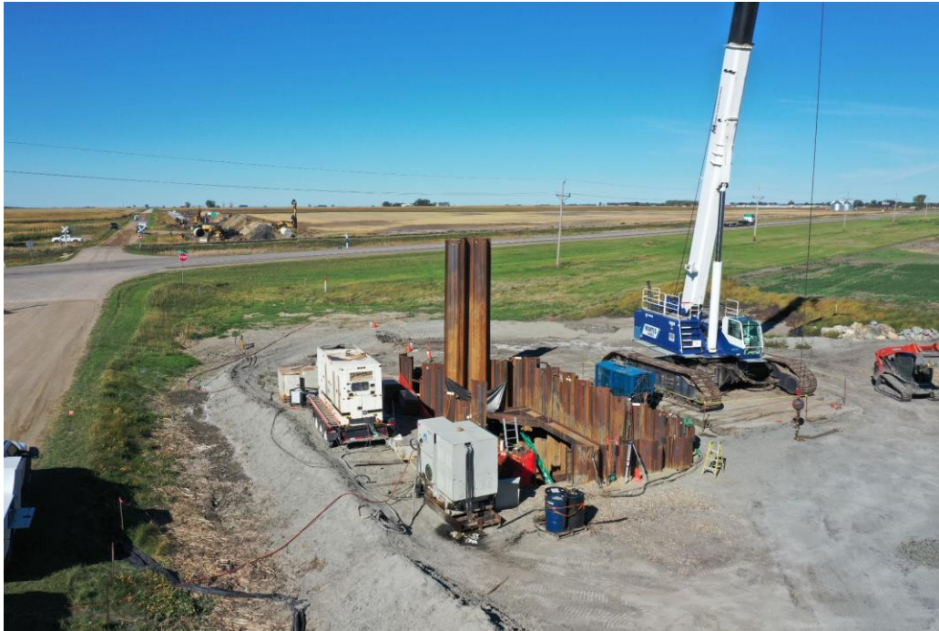
Figure 5 RRVWSP 72-inch Trenchless Crossing Launching Shaft
