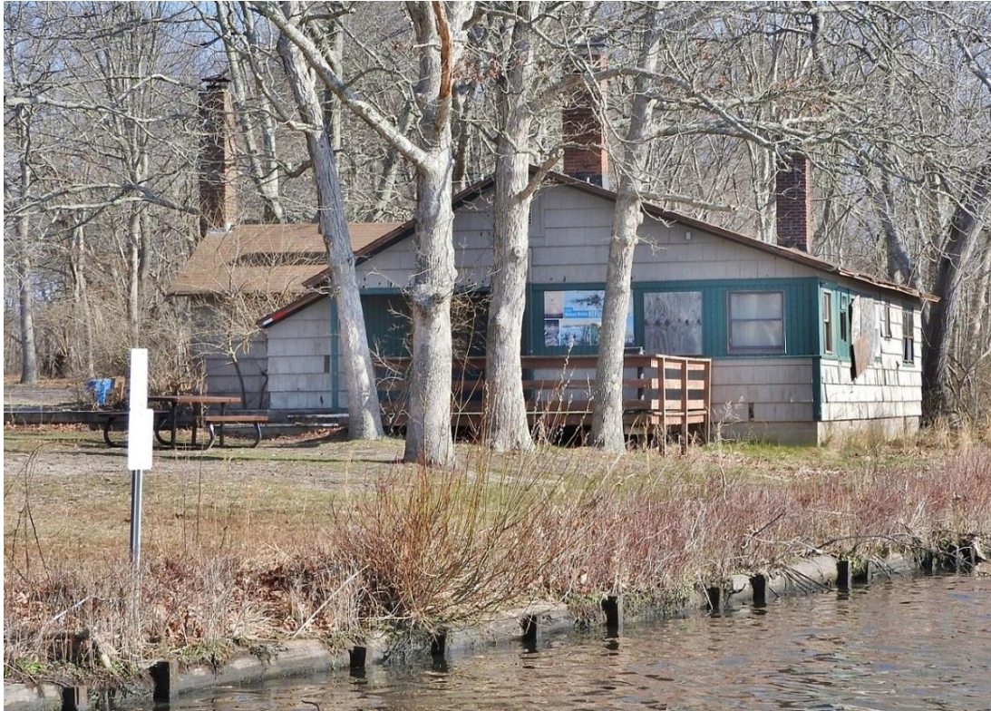
5. Facing north toward Cabin.
