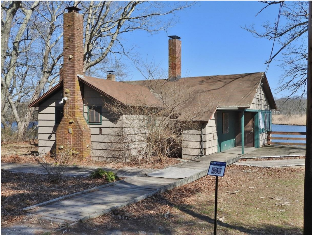
11. Facing east toward west wing and main block.
