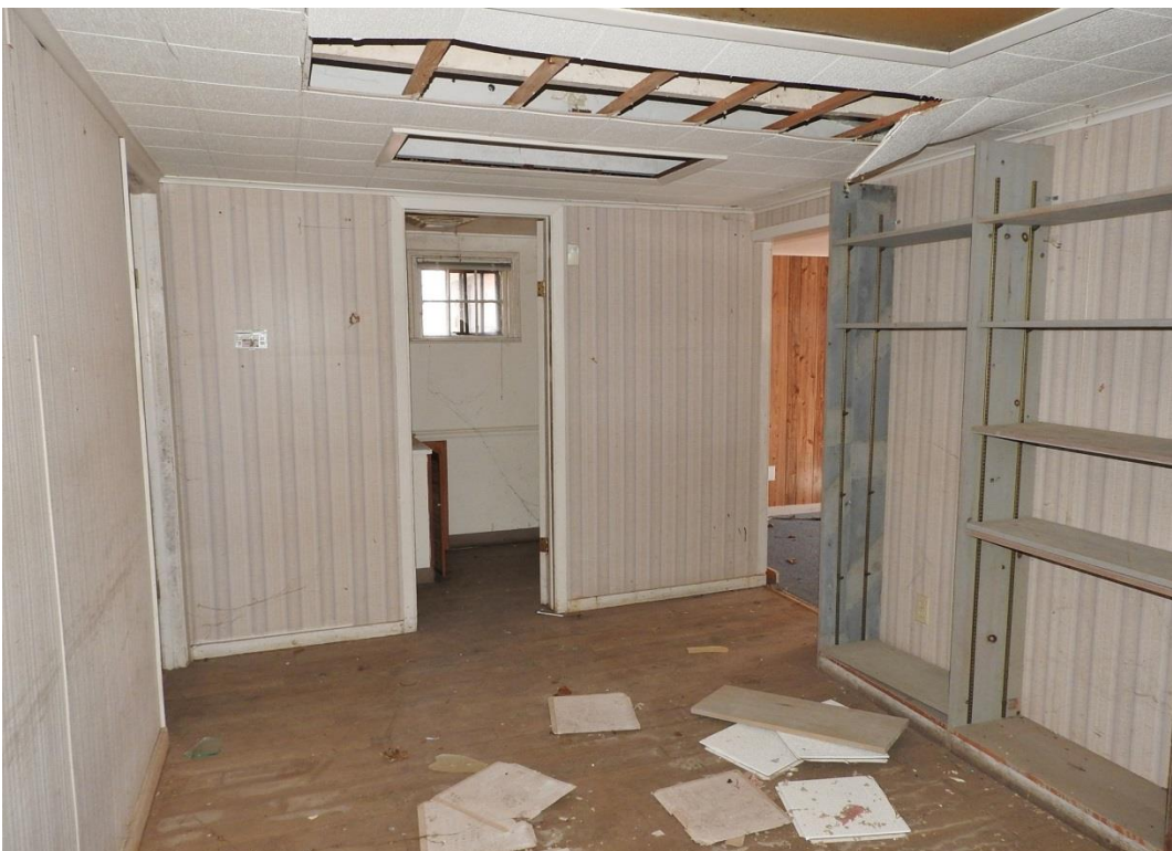
22. Facing northeast in west room of main block.
