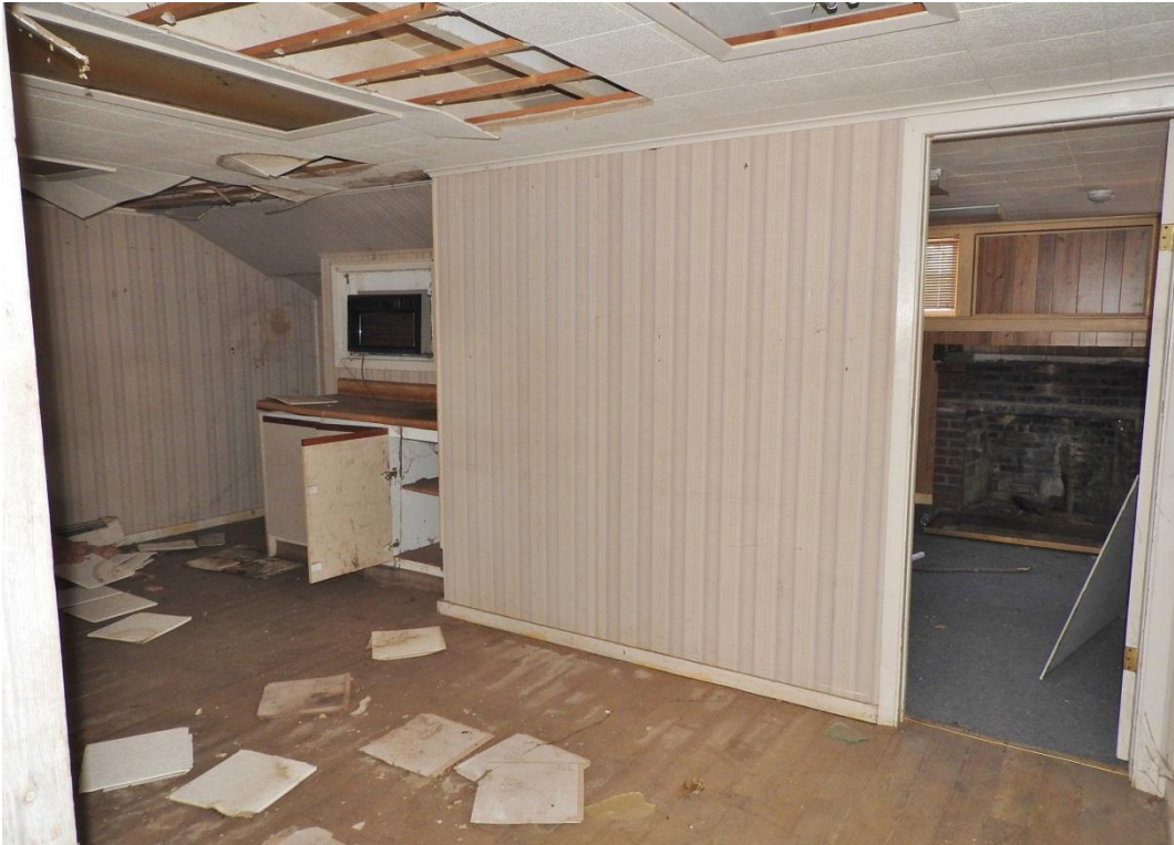
21. Facing southwest in west room of main block.
