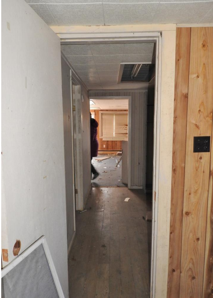
23. Facing east from west room of west wing into main block.
