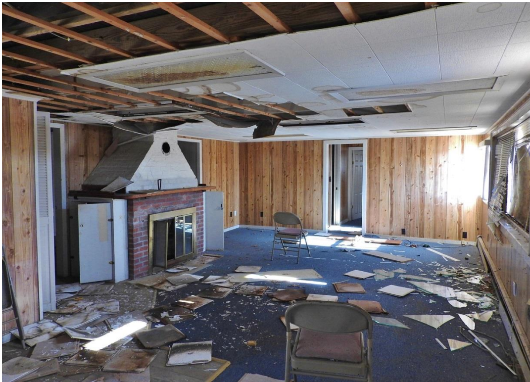
17. Facing north in main block.
