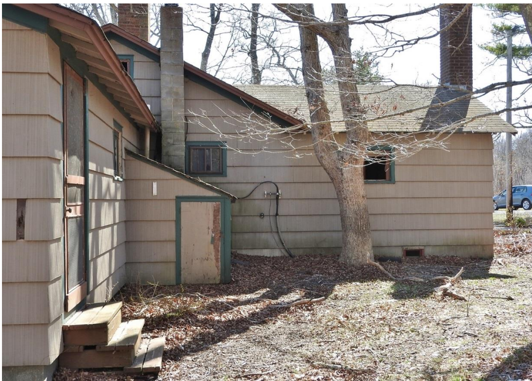
16. Facing south toward north wing, main block, and west wing.
