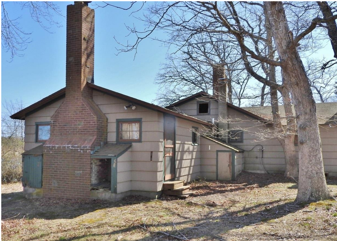
13. Facing south toward north wing.
