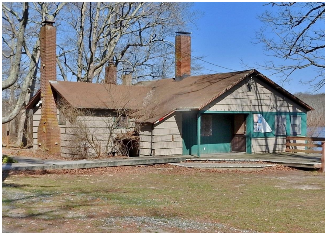
7. Facing northeast toward west wing and main block.
