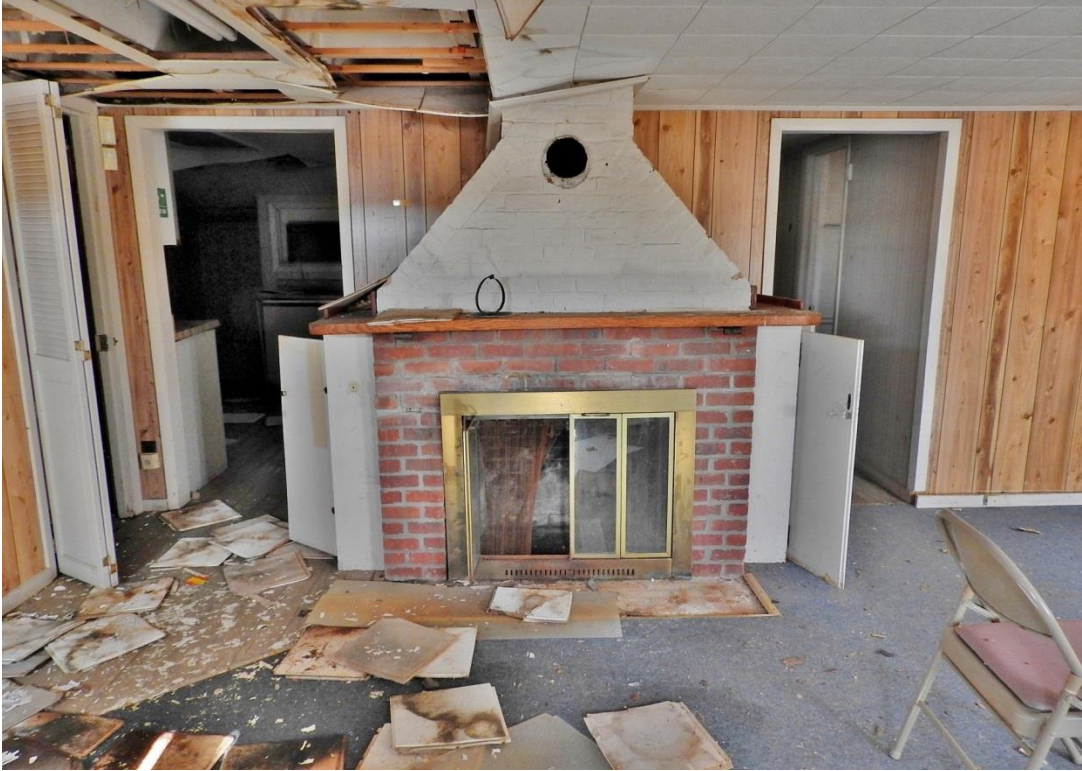
19. Facing west in main block.
