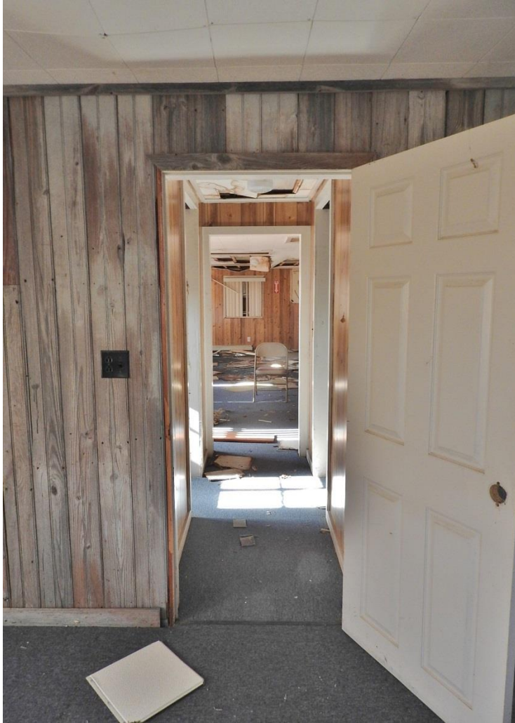
28. Facing south from north room of north wing into main block.
