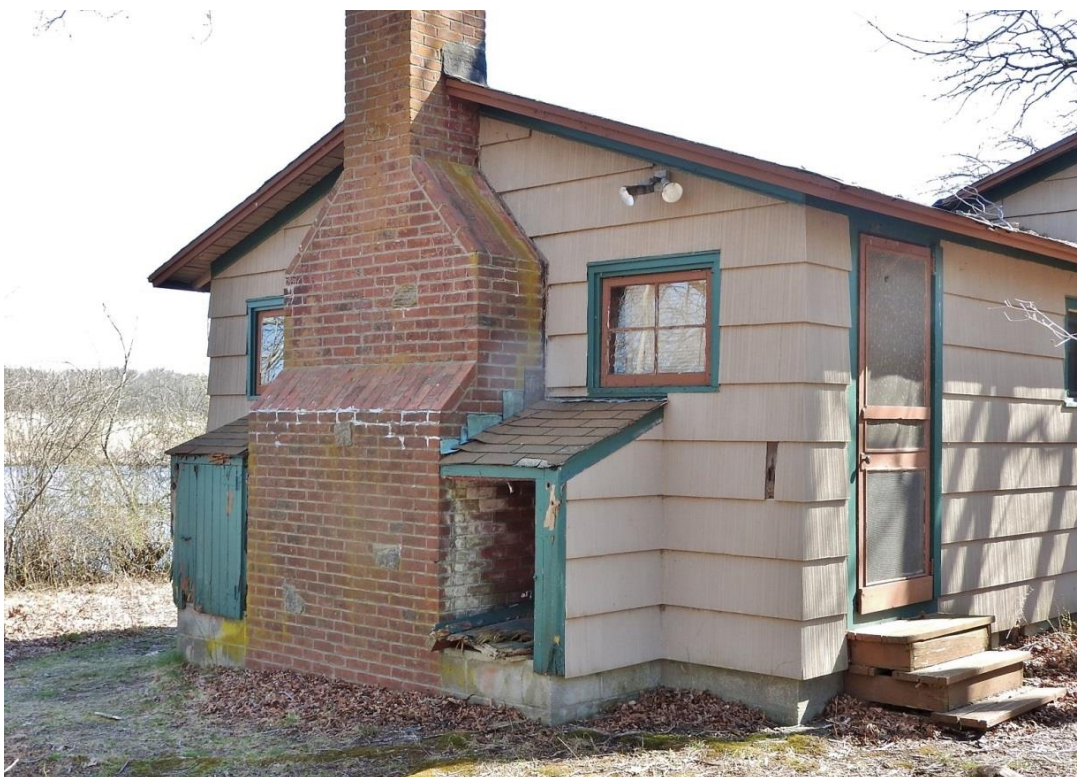
14. Facing southeast toward north wing.
