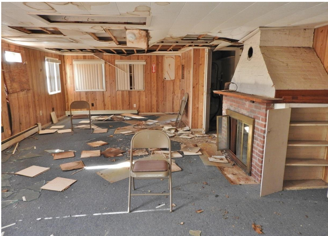
18. Facing south in main block.
