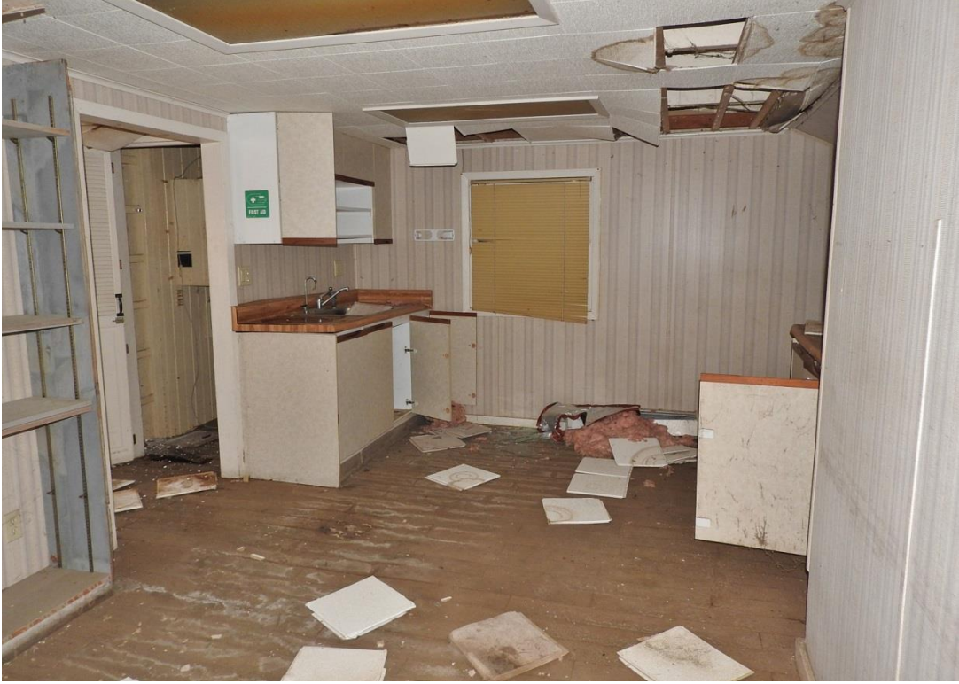
20. Facing south in west room of main block.
