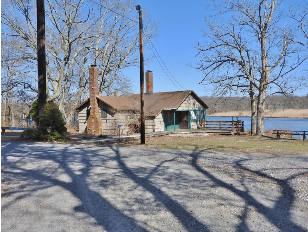
3. Facing east toward Cabin across service road.
