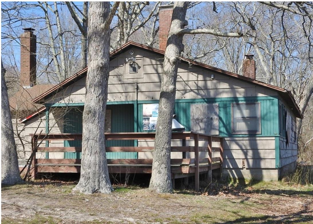
6. Facing north toward main block and front (south) elevation.
