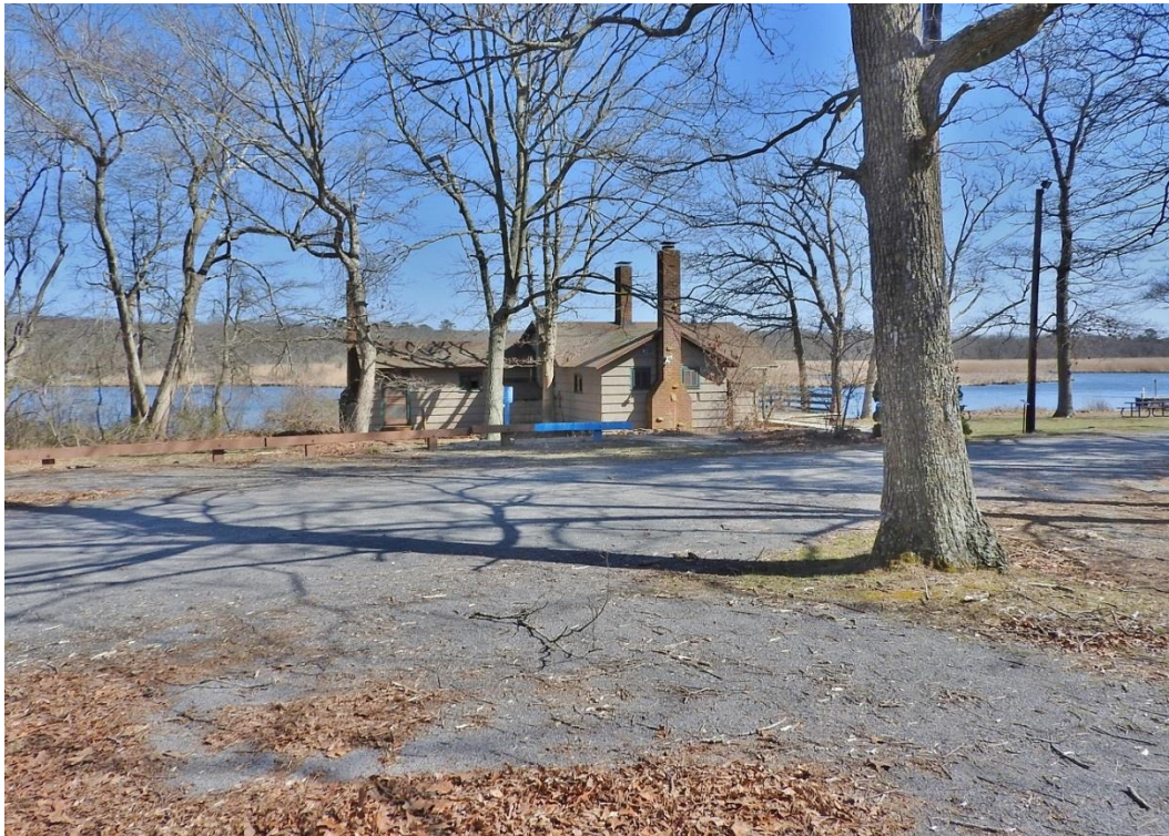
4. Facing southeast toward Cabin across service road.
