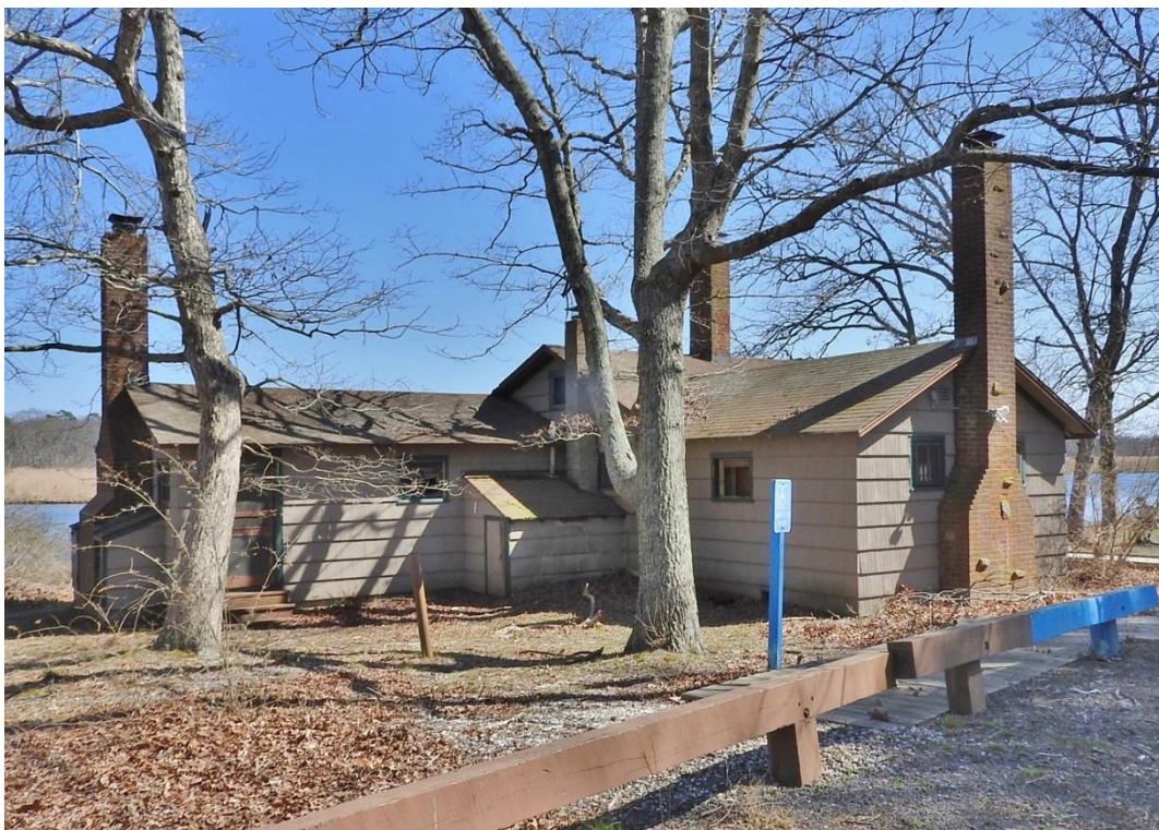
12. Facing southeast toward north wing and west wing.
